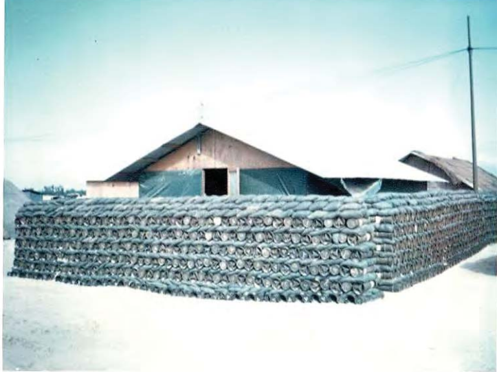
Blast wall around a hootch
